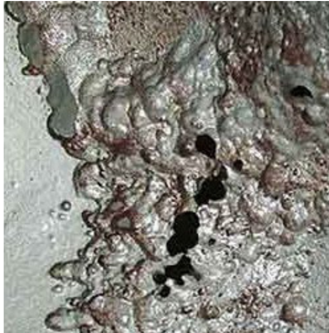
Severe (through wall) cavitation damage to metallic components
